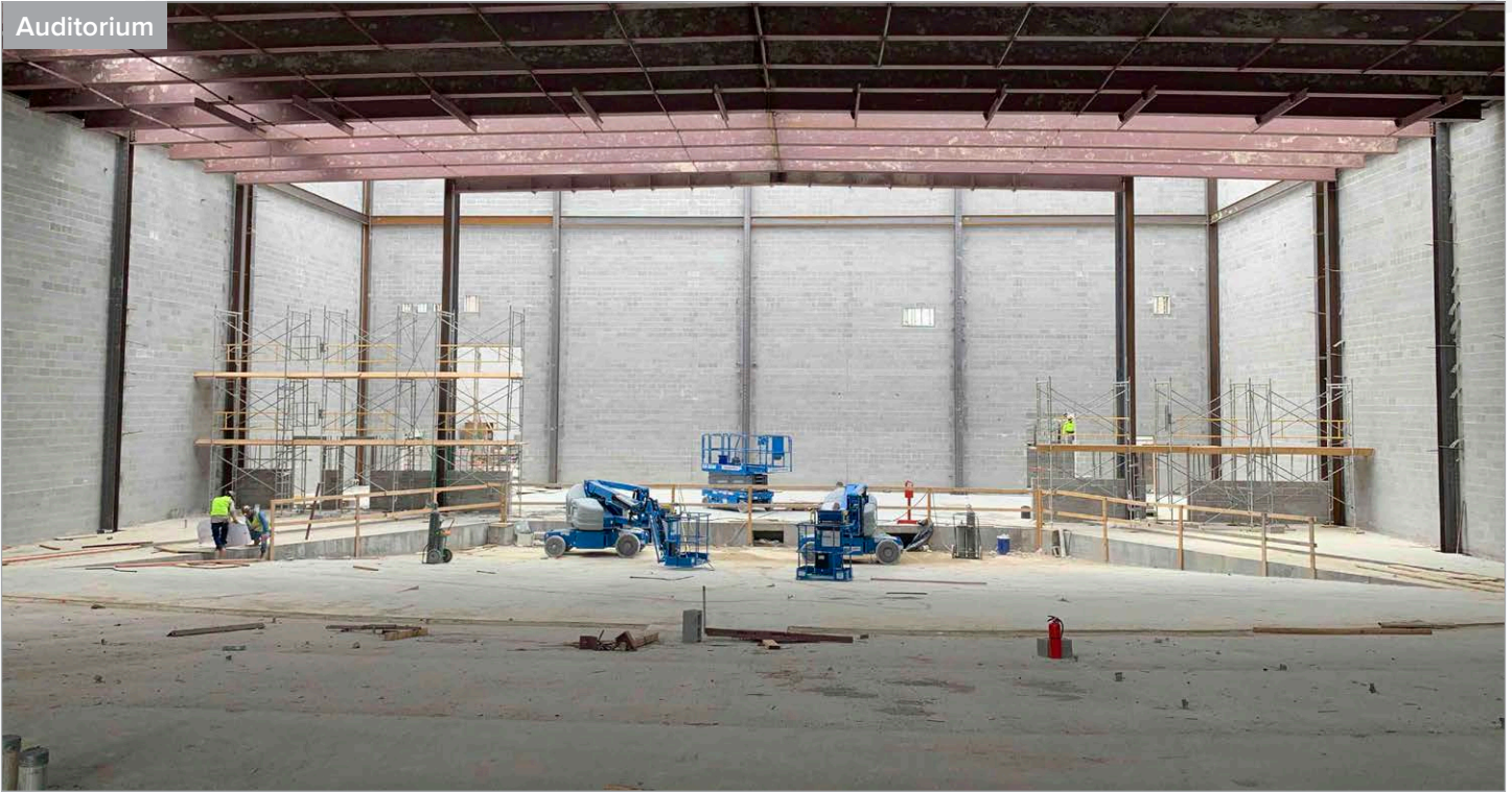
Auditorium Structural Steel and Roof Deck
